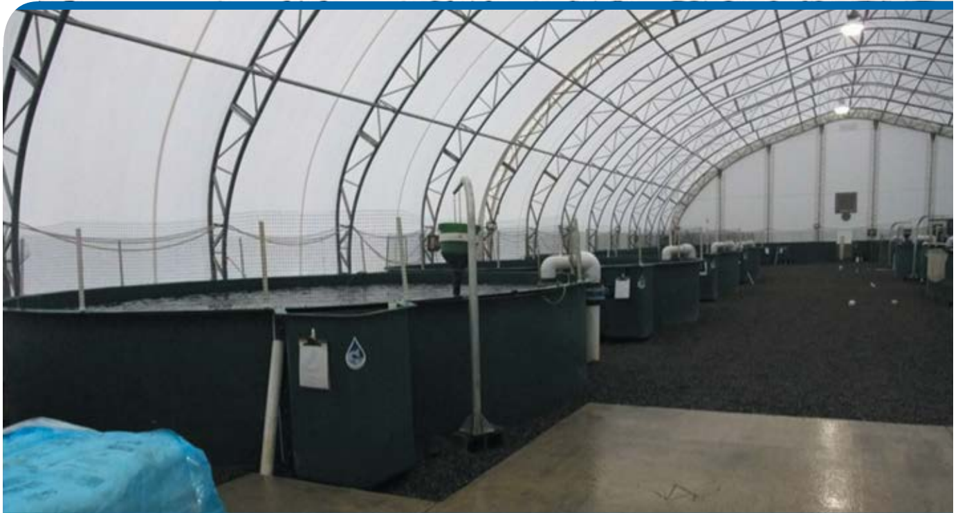
Senators toured Taste of BC Aquafarms Inc., a small family business operating a land-based closed-containment facility in Nanaimo, which utilizes 15 different tanks. The company raises Steelhead salmon using recirculating aquaculture systems.
